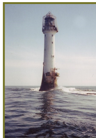
Bell Rock Lighthouse
