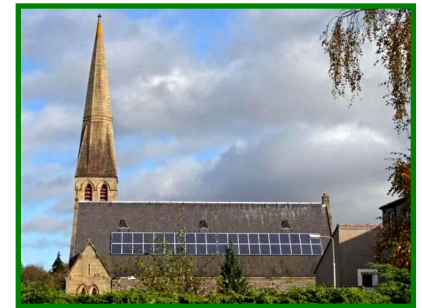
INSTALLING SOLAR PANELS & LOW CARBON HEATING Image: David Bethune, used with permission
