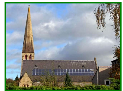
INSTALLING SOLAR PANELS & LOW CARBON HEATING Image: David Bethune, used with permission
